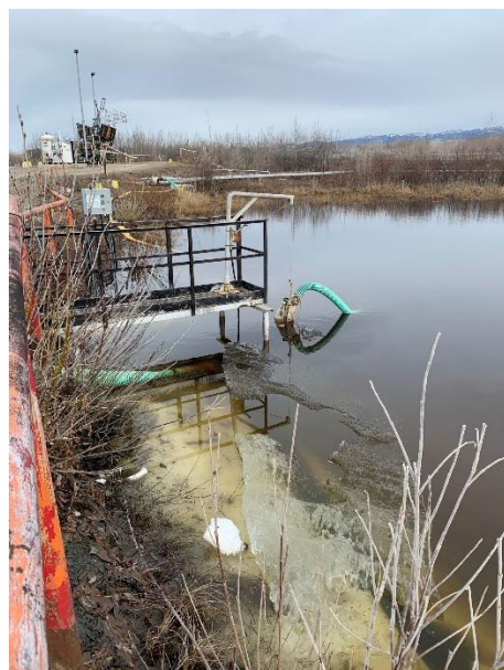
Figure 5-2: Refinery Impound Basin Elevated Volumes Event After Discharge
