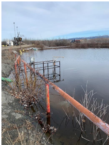
Figure 5-1: Refinery Impound Basin Elevated Volumes Event Before Discharge
